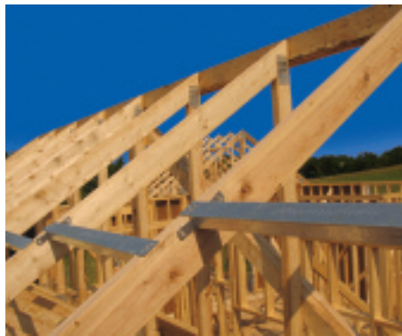
The Stabilizer spaces and braces in one step with just a hammer.
